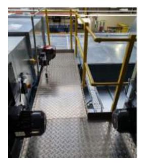
As Part of the project, we installed access walkaways to ensure that plant service and maintenance can be carried out easily and safely.
